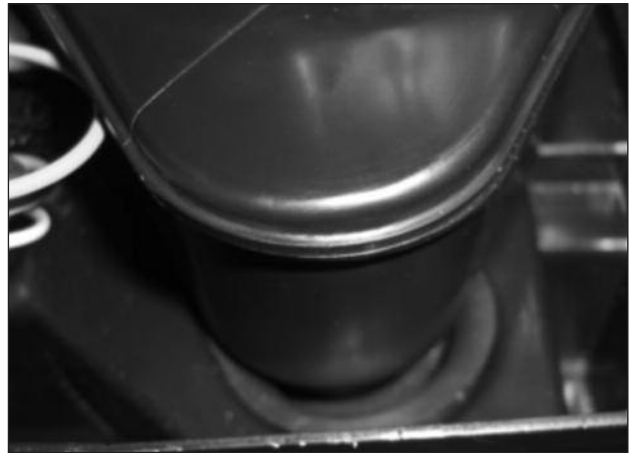
Fig. 9: Proper Engagement of Condensate Pan
